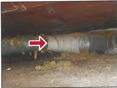
Apparent asbestos material
