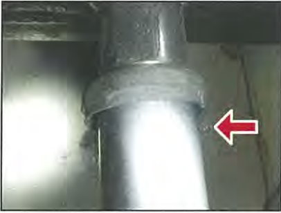
Leaking drain piping
