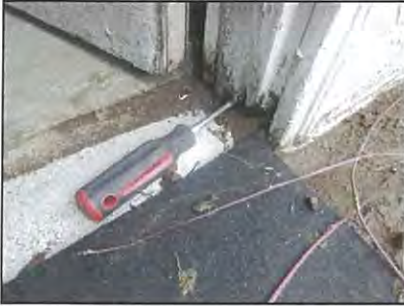
Damaged door & frame
