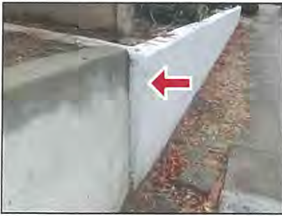
Leaning retaining wall
