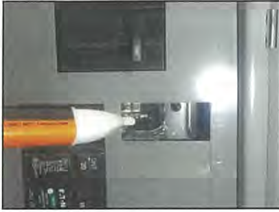
Missing twist-out
