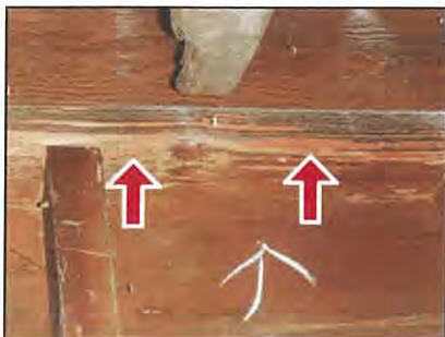
Damaged cripple walls
