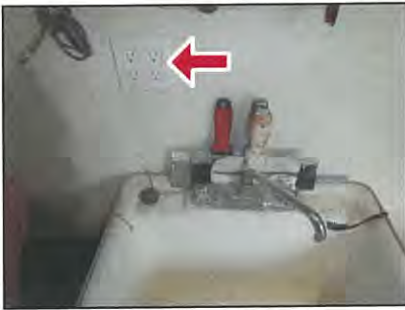
Unsafe outlets near sink
