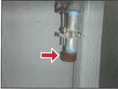
Corroded gas piping
