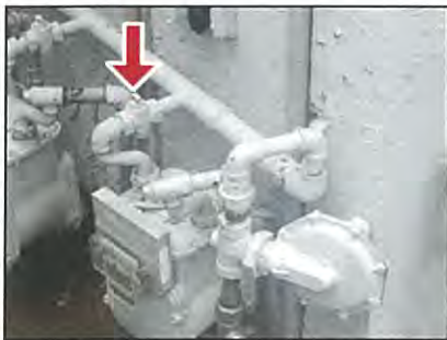
Main gas shutoff valve
